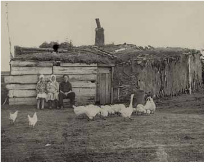
Rear view of a one-room hovel in Novosibirsk oblast. An animal shelter is on the right, and the entrance is on the left. Visible in the wall are sticks and twigs used in the construction. Building materials had to be scavenged.
